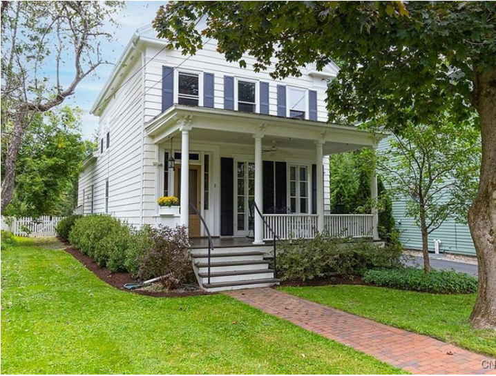
3 Nickerson St, 2 nd Floor Window Replacements
